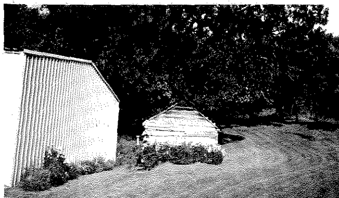
The old and the new—1872 log cabin that John Walla built when he homesteaded. Steel building built by the Groffs in 1981. Jean Groff is the great granddaughter of John Walla.
