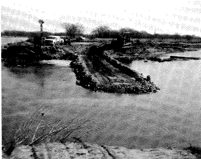
Repairing the dike, 1978
