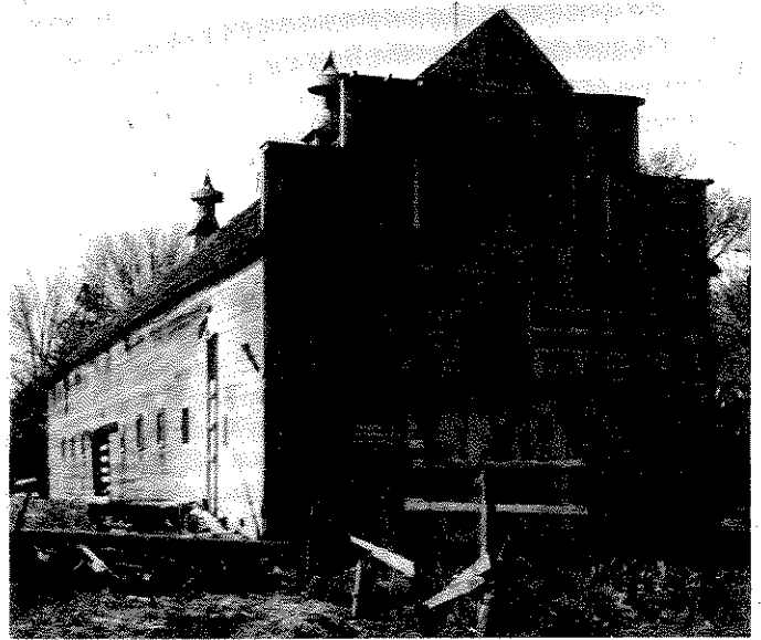
This huge livery barn was originally located at 2nd & Short Streets.
