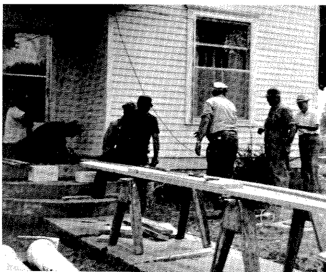
Work on the rectory by men of both parishes.
